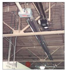
The inside of the test site, representing a typical industrial building and showing the RE-VERBER-RAY Two-Stage *HL Series*. This heating system objectively documented a minimum of 12% additional energy savings - and a 35% reduction in "On and Off Cycles" - when compared to a single input system.
