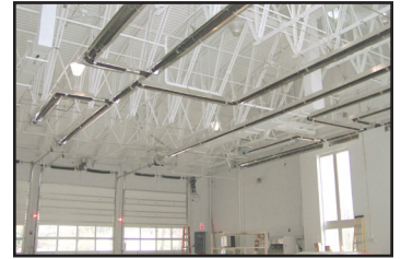
Fire Station Apparatus Bays
